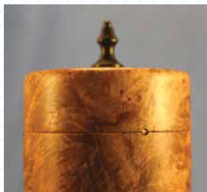
An unobtrusive pin affixed at the box/lid juncture registers the lid at the correct grain orientation.
